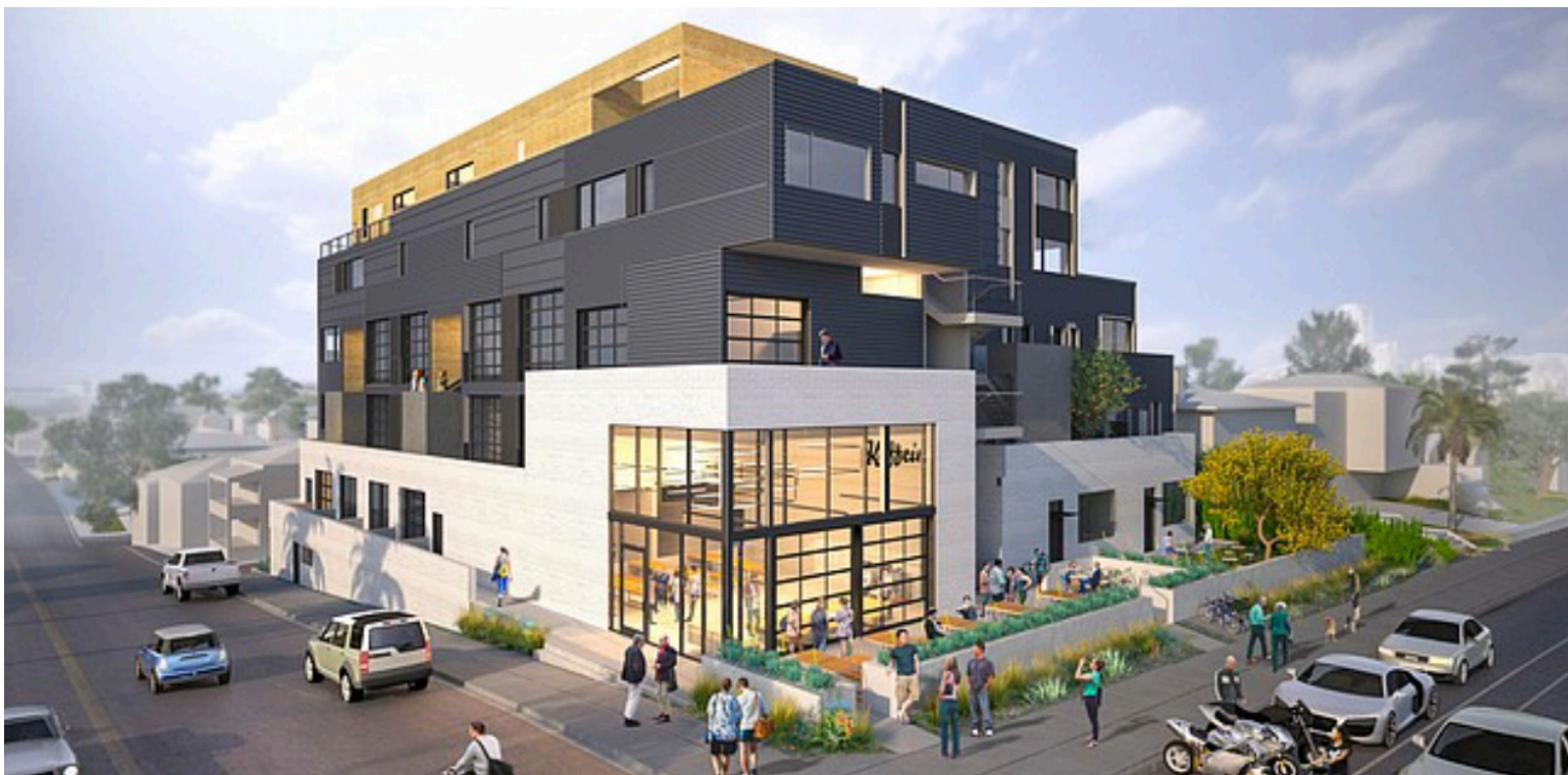
Buzz is a $9 million apartment project under construction on the east side of I-5 in Golden Hill. Rendering courtesy of Rammy Urban Infill and Hub & Spoke Communities.
